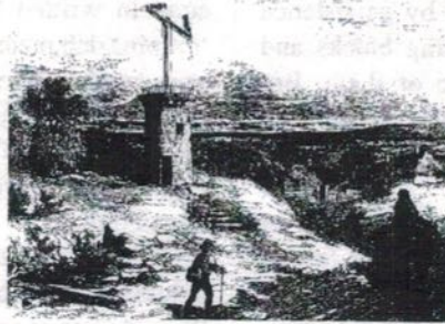
A repeater station on the North line
