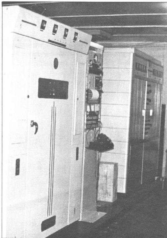
First replacement of ANARE war surplus transmitting equipment. (On left) Philips 1619C one kilowatt transmitter at Mawson. On right, a CTH7 5 kw transmitter of later vintage.
