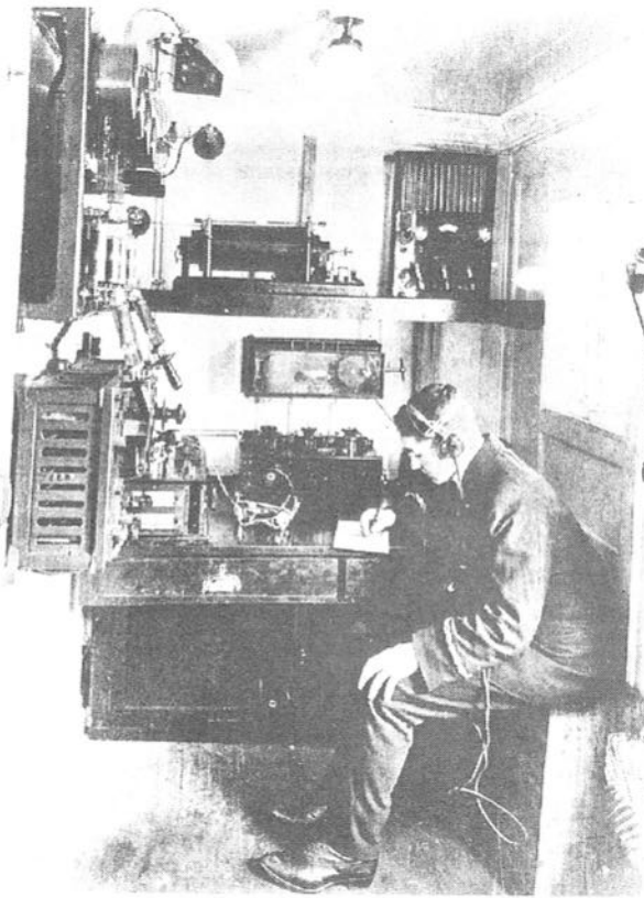
The Standard Ship Radio Room: This is thought to be the radio room (or Marconi room) on the Cunard passenger ship Carpathia, which went to the rescue of the Titanic, with Harold Cottam, the radio officer involved. The magnetic detector and multiple tuner are to his right, with the emergency spark transmitter on the shelf above. The Marconi valve receiver is on the table to the left, partly obscured by the casing of the motor and alternator starters. The high resistance headphones for the valve receiver are on the table and he appears to be using the magnetic detector!
