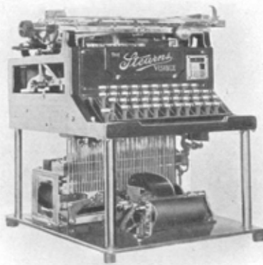
Burlingame Telegraphing Apparatus Attached To a "Stearns" Typewriter
