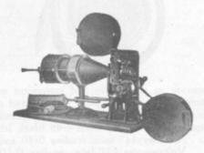
When used with the arc light, the projector will give brilliant screen pictures 3 x 4 feet at a distance of 12 feet, 4 x 5 feet at 15 feet, and 5 x 7 feet at 20 feet, and larger pictures at a greater distance with but slight decrease in brilliancy.
